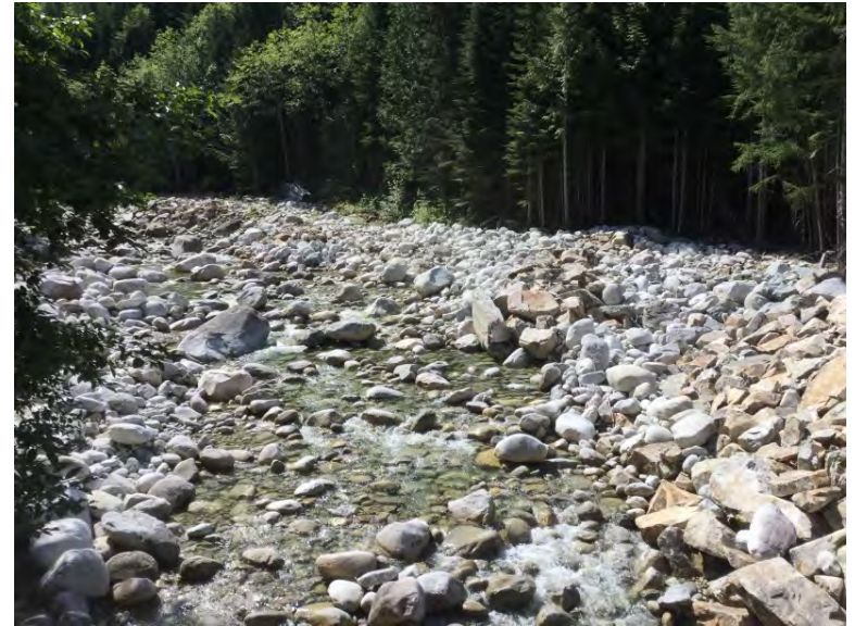
Groins upstream left bank
