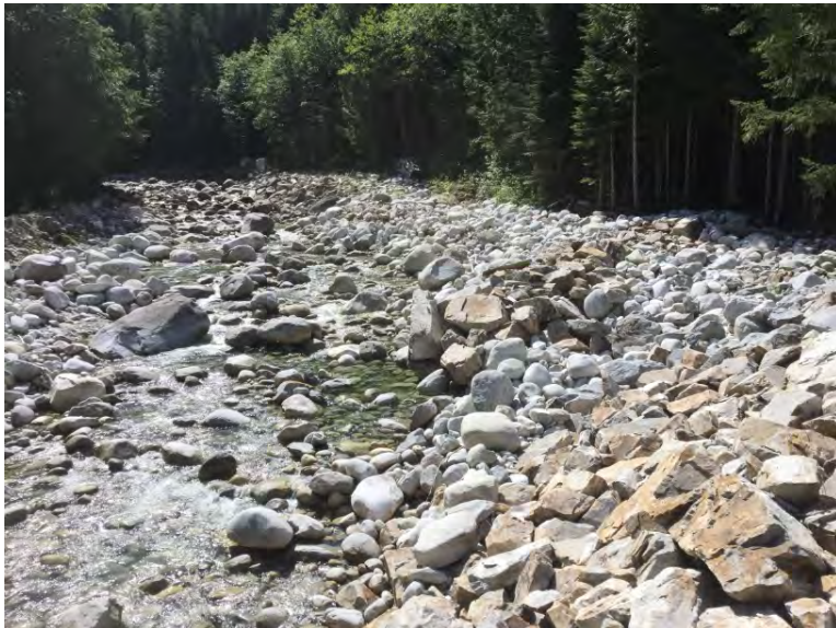
Groins upstream left bank
