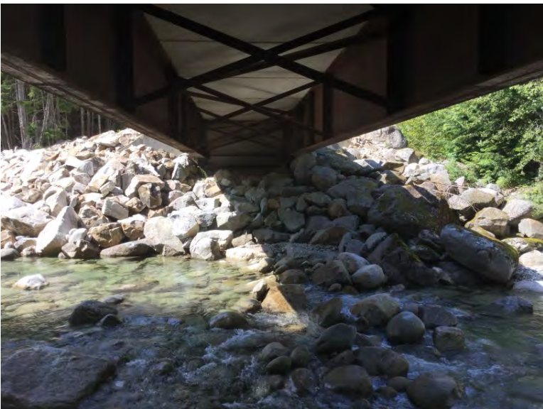
Left Bank Abutment when facing downstream
