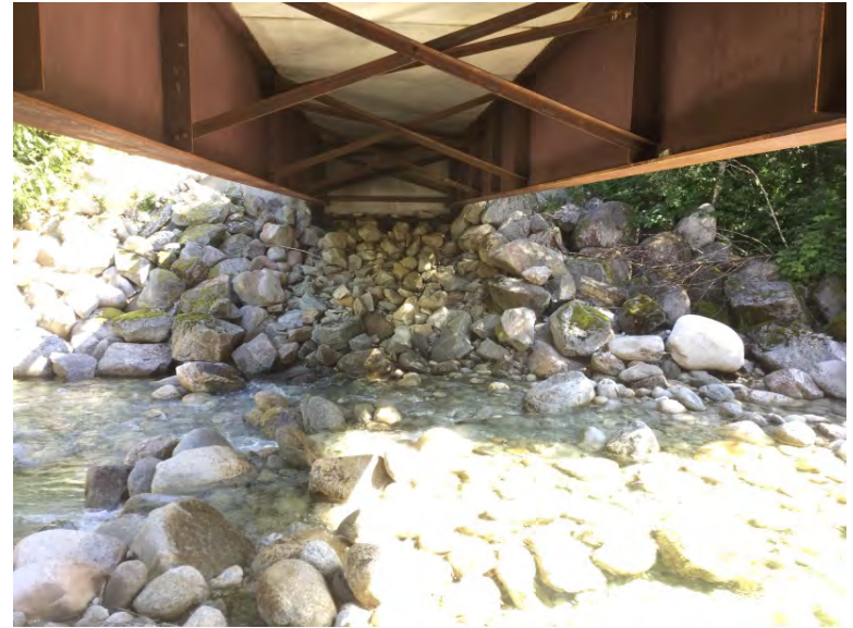
Right Bank Abutment when facing downstream
